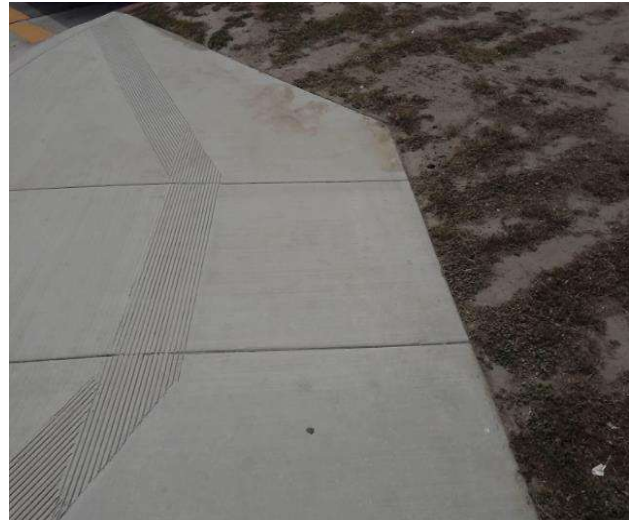
Curb Ramp , Landings and Transitions : Bottom Landing Of Diagonal Curb Ramp - Clear Space
