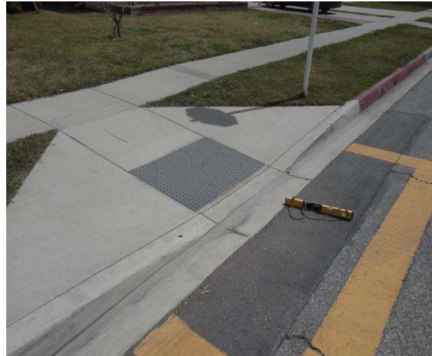
Curb Ramp : Bottom Landing Slope
