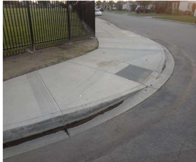
Curb Ramp : Bottom Landing Slope
