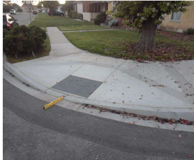
Curb Ramp : Bottom Landing Slope
