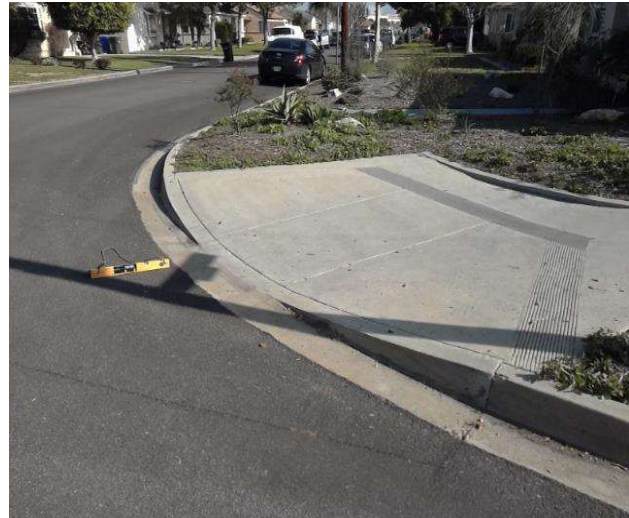
Curb Ramp : Bottom Landing Slope
