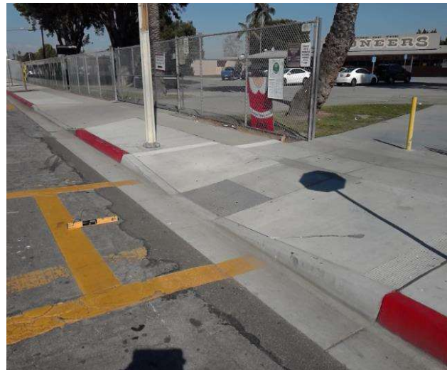
Curb Ramp : Bottom Landing Slope
