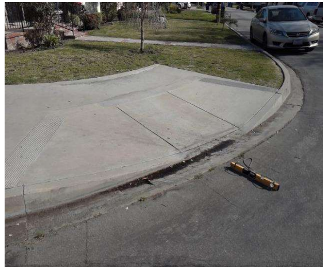
Curb Ramp : Bottom Landing Slope
