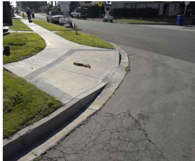
Curb Ramp : Bottom Landing Slope
