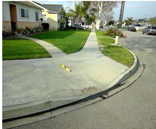
Curb Ramp : Bottom Landing Slope
