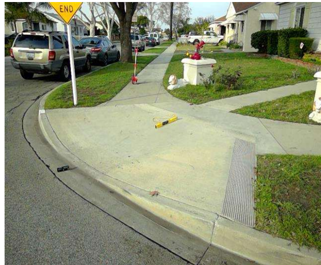
Curb Ramp : Bottom Landing Slope
