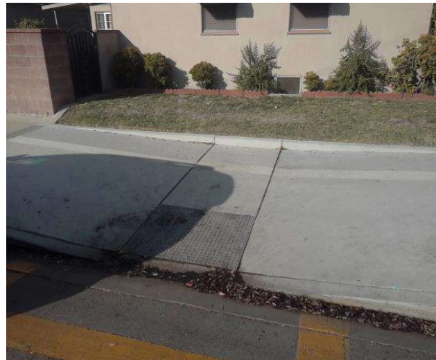
Curb Ramp : Bottom Landing Slope
