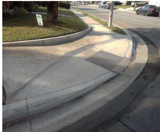
Curb Ramp : Bottom Landing Slope
