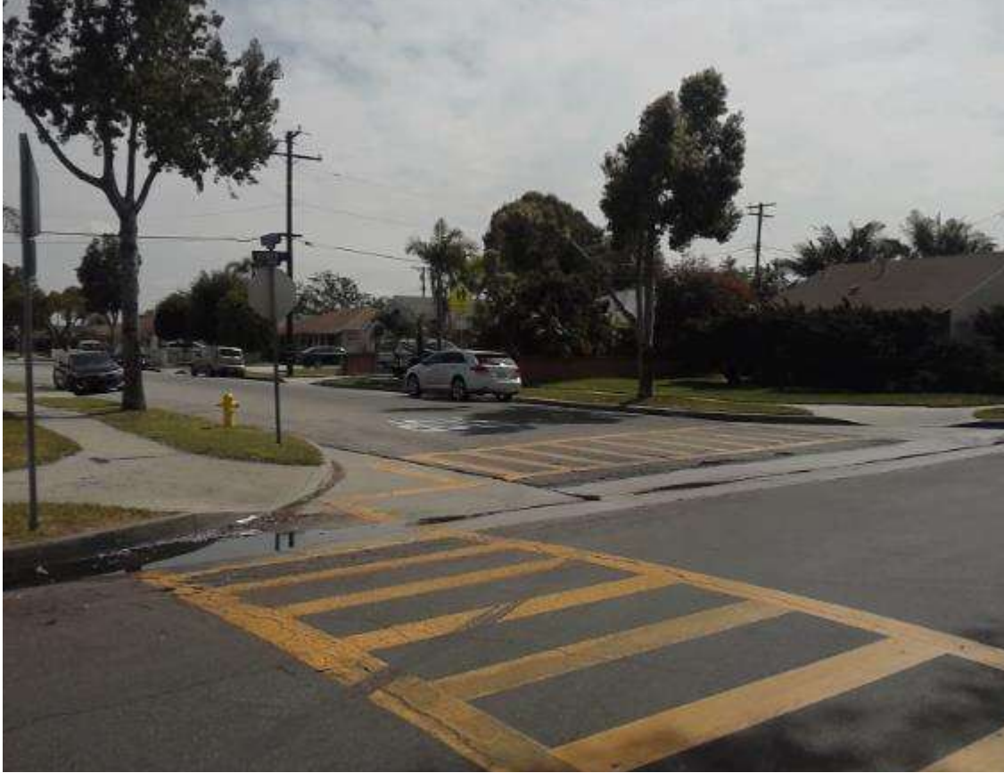
Julius Avenue - Adwen Street To Pivot Street
