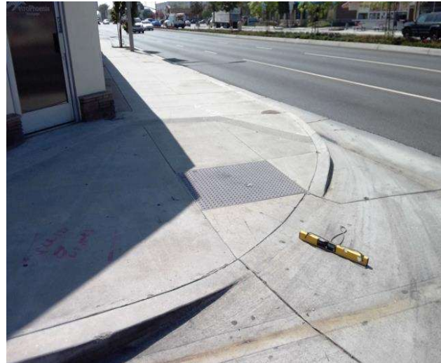
Curb Ramp : Bottom Landing Slope
