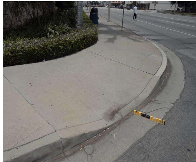
Curb Ramp : Bottom Landing Slope
