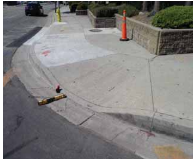
Curb Ramp : Bottom Landing Slope
