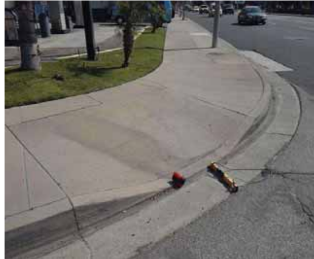
Curb Ramp : Bottom Landing Slope
