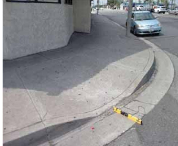
Curb Ramp : Bottom Landing Slope
