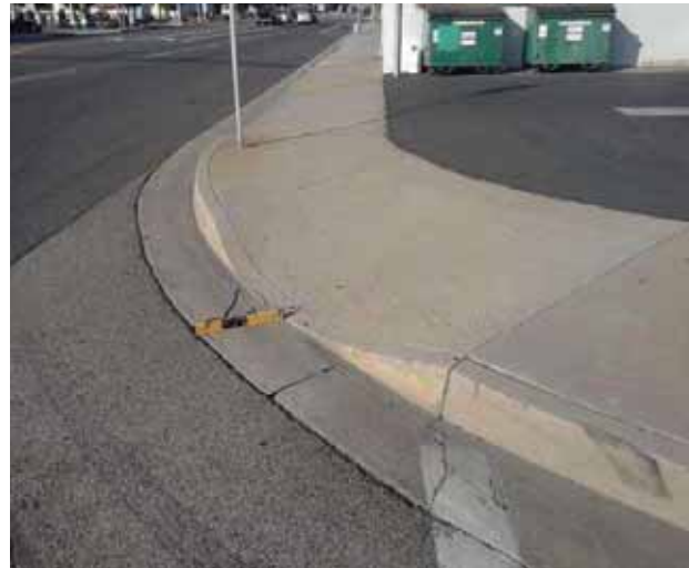
Curb Ramp : Bottom Landing Slope
