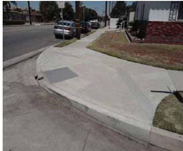
Curb Ramp : Bottom Landing Slope
