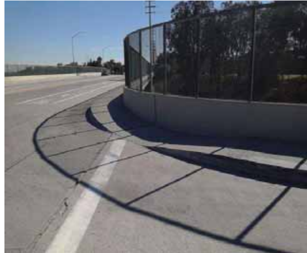
Curb Ramp , Landings and Transitions : Top Landing Right Side Slope - Parallel Curb Ramp
