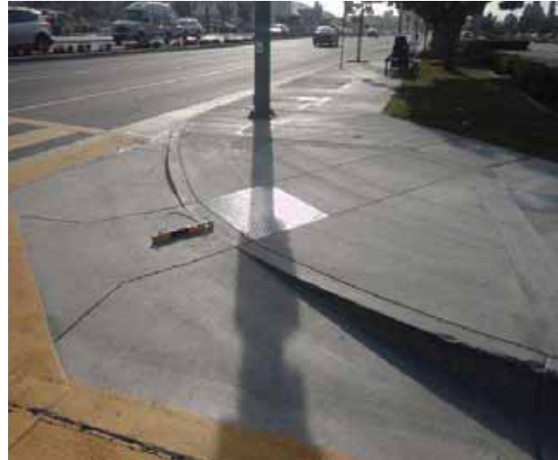
Curb Ramp : Bottom Landing Slope
