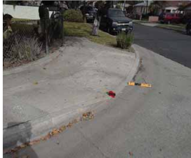
Curb Ramp : Bottom Landing Slope
