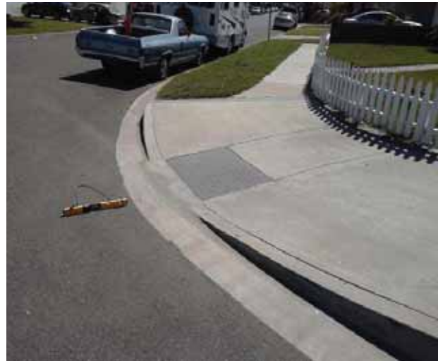
Curb Ramp : Bottom Landing Slope
