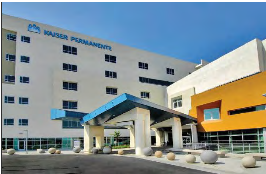
Figure 2-1: Kaiser Permanente Downey Medical Center, 9333 Imperial Highway
