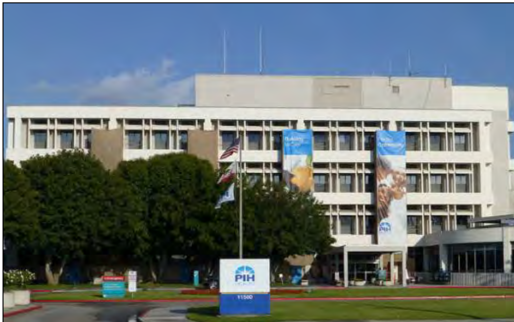
Figure 1-1: PIH Health Hospital, a non-profit community hospital located within Downey's Hospital/Medical Arts Zone, 11500 Brookshire Avenue
