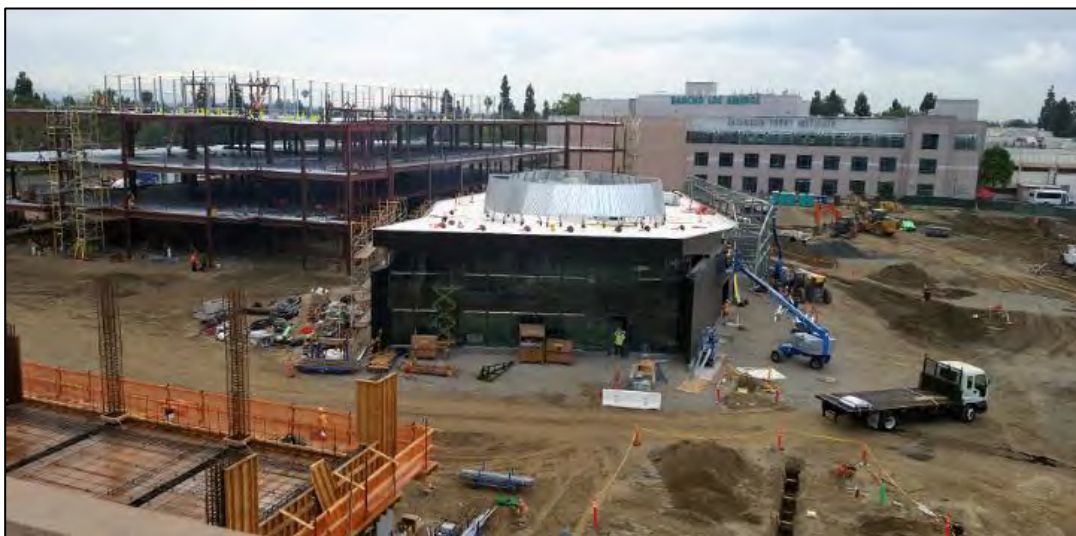
Figure 2-3: Rancho Los Amigos National Rehabilitation Center, major remodel and expansion, 2016
