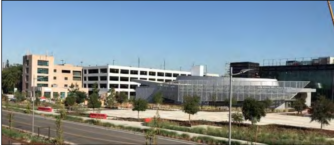
Figure 2-2: Portion of Rancho Los Amigos National Rehabilitation Center, 7601 East Imperial Highway
