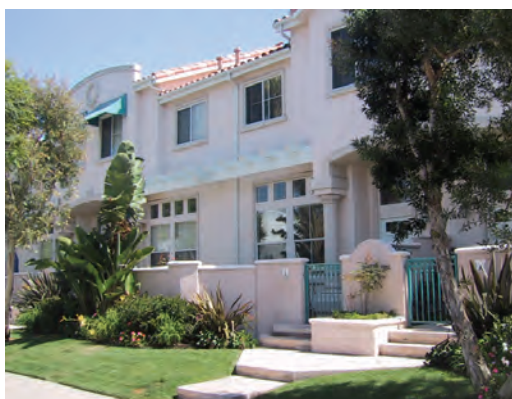
Image (bottom): Pedestrian entries are emphasized through stoops and overhangs at entries.
