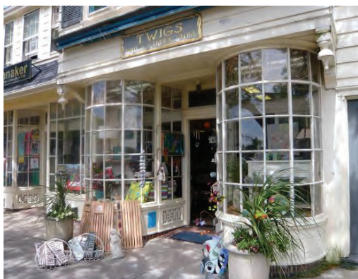
Image (top): Details shown here include recessed entries, bay windows, mullions, and moldings.
