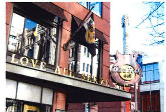
D. Hybrid sign. Combines canopy pan-channel with 3D fabricated object incorporating various signage elements.
