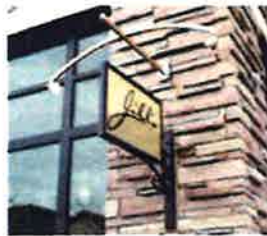
Externally illuminated faux painted sign panel
