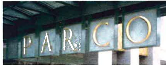
Prismatic gilded letters mounted to a glass substrate
