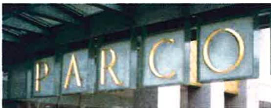
Prismatic gilded letters mounted to a glass substrate
