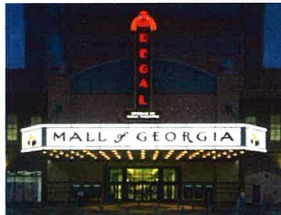
Internally illuminated marquee with exposed neon vertical sign.
