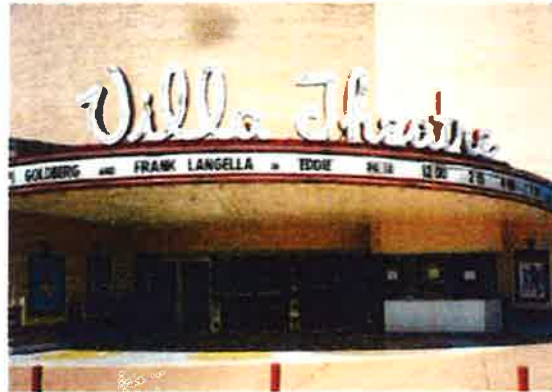
Freestanding exposed neon letters on marquee canopy.
