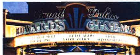
Internally illuminated marquee with edge illuminated pan channel letters.
