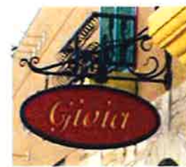
Externally illuminated with incised and gilded type
