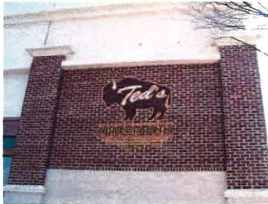
A. Wall painted graphic with Tenant name or logo. To be included in total square footage.
