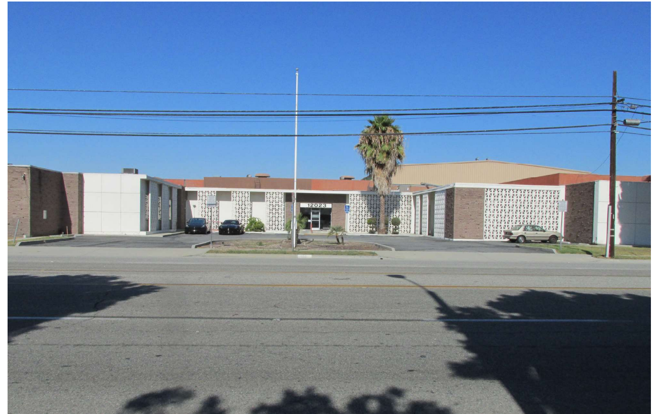
Photograph B View of the Project Site looking east from Woodruff Avenue towards the front office.
