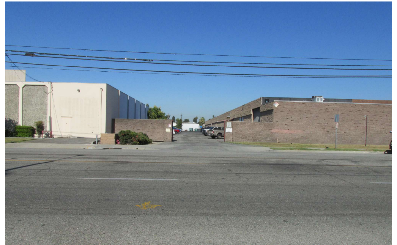
Photograph D View of the Project Site looking east from Woodruff Avenue towards Driveway 2.
