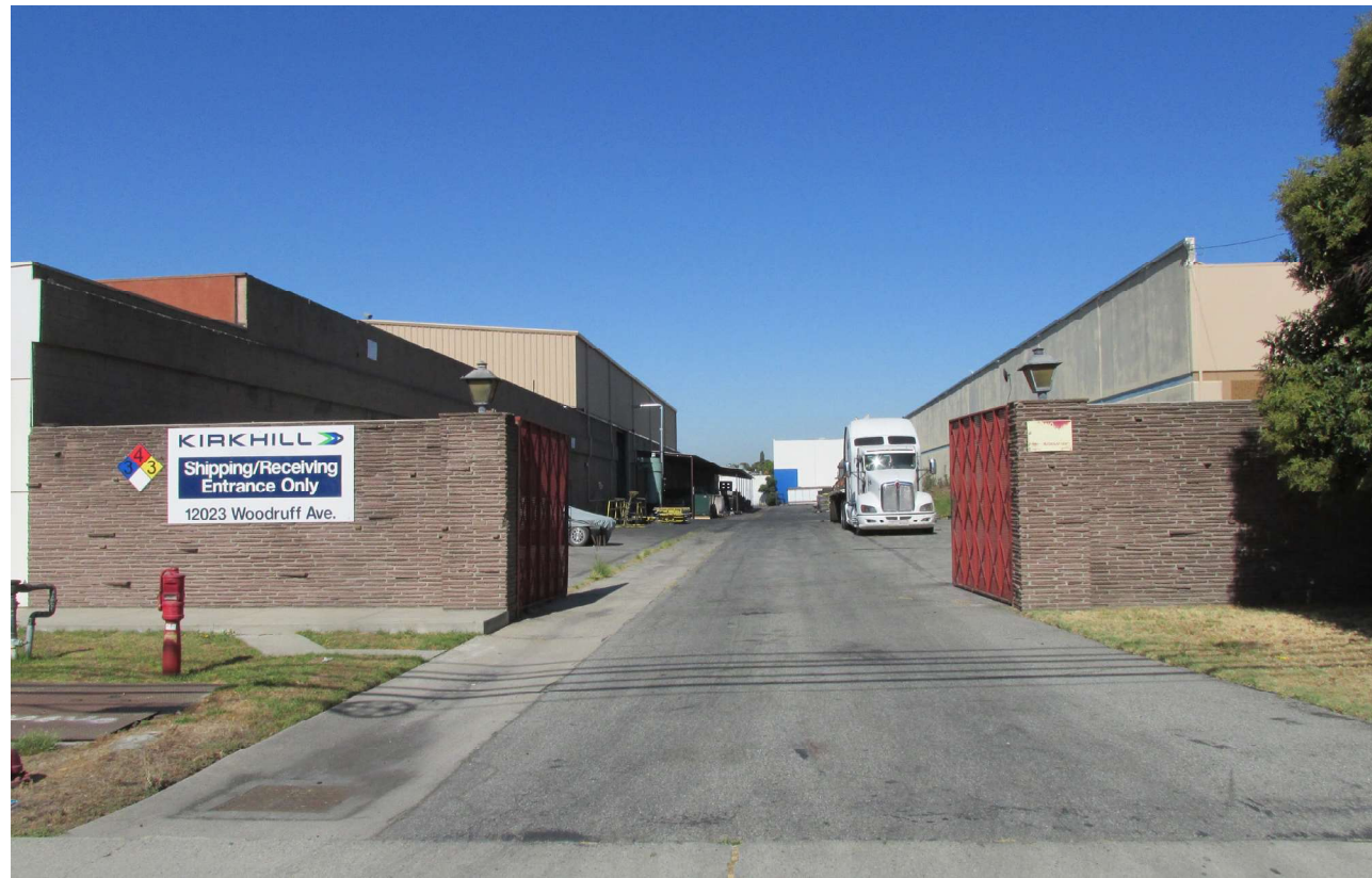
Photograph C View of the Project Site looking east from Woodruff Avenue towards Driveway 1.
