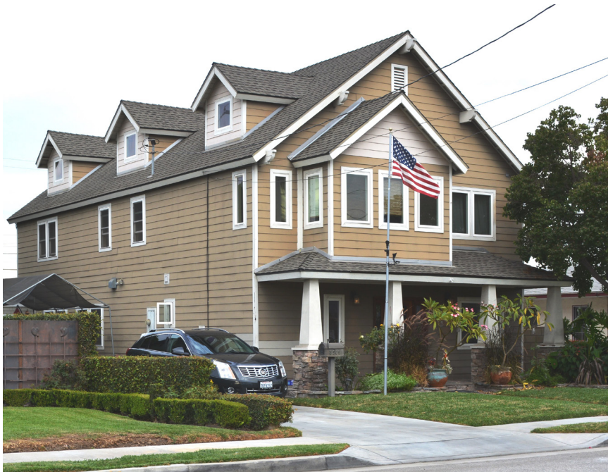
FIGURE 28: Side-facing windows at second stories should not exceed fifteen (15) percent of the aggregated side yard-facing façade area.
