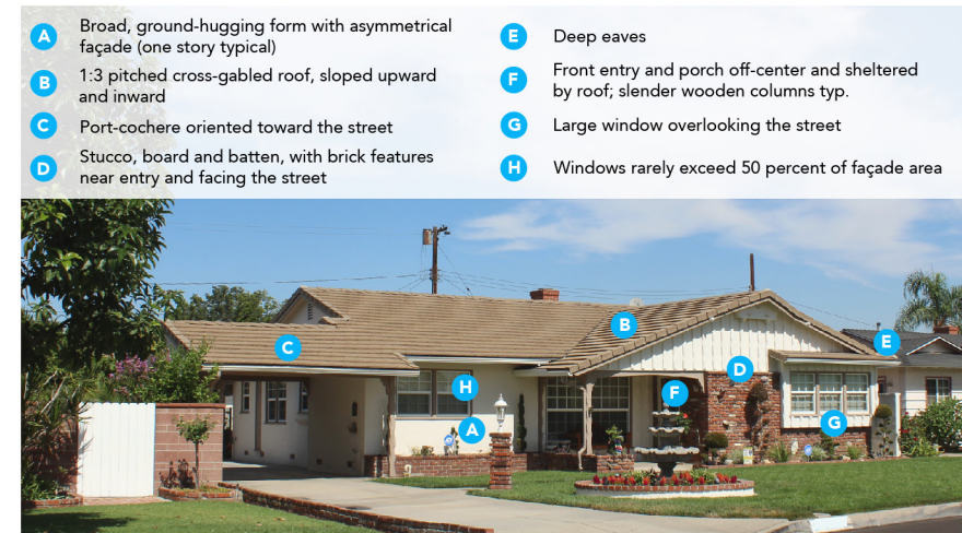
FIGURE 2: Ranch Style (Note: Porte-cocheres are subject to setback standards per Section 9312.08 of the Downey Municipal Code)
