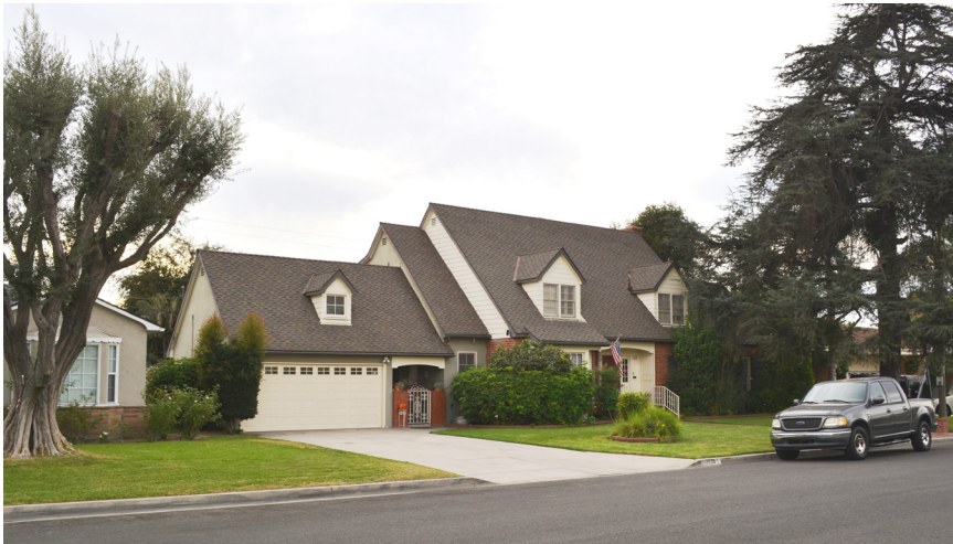
FIGURE 24: This home utilizes single-story characteristics such as incorporating dormers and encasing the first and second story under a singular roof.
