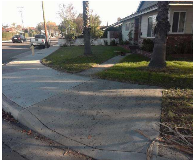
Curb Ramp : Bottom Landing Slope
