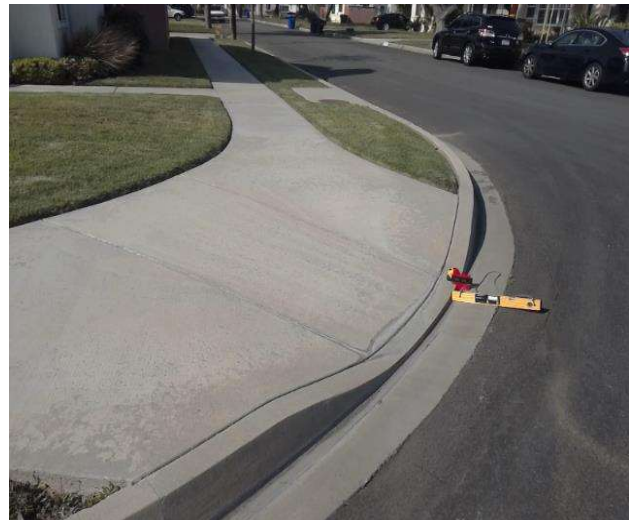
Curb Ramp : Bottom Landing Slope
