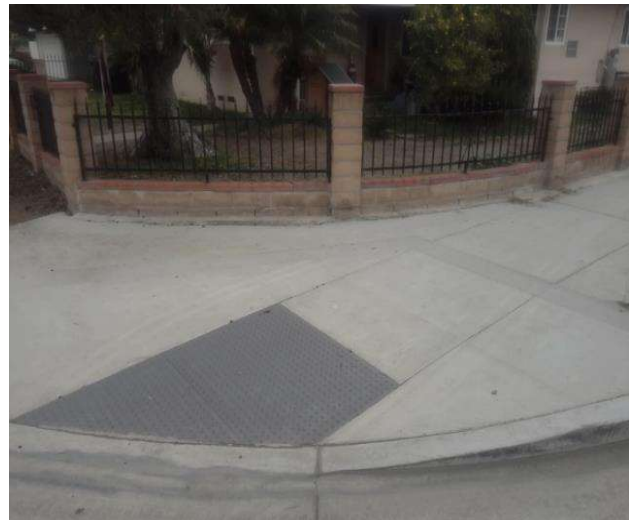
Curb Ramp : Bottom Landing Slope
