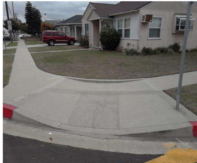
Curb Ramp : Bottom Landing Slope
