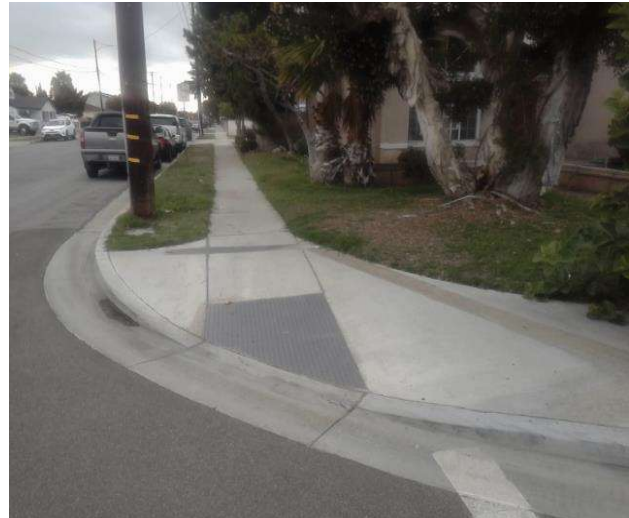
Curb Ramp : Bottom Landing Slope
