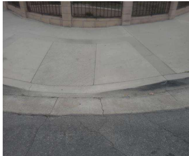
Curb Ramp : Bottom Landing Slope
