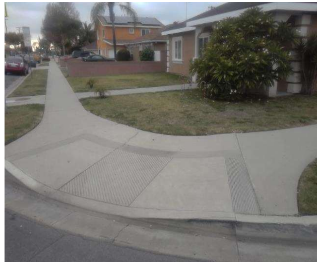
Curb Ramp : Bottom Landing Slope
