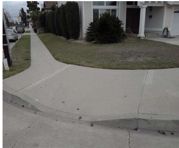
Curb Ramp : Bottom Landing Slope
