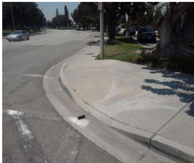
Curb Ramp : Bottom Landing Slope
