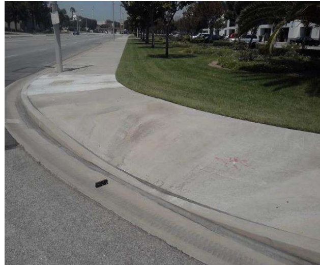
Curb Ramp : Bottom Landing Slope
