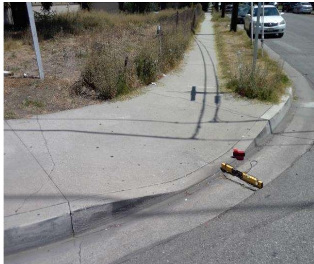
Curb Ramp : Bottom Landing Slope
