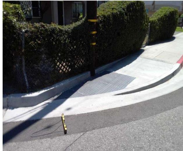
Curb Ramp : Bottom Landing Slope
