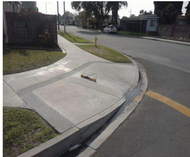
Curb Ramp : Bottom Landing Slope
