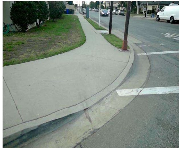
Curb Ramp : Bottom Landing Slope
