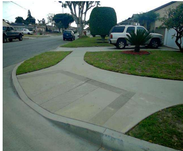
Curb Ramp : Bottom Landing Slope
