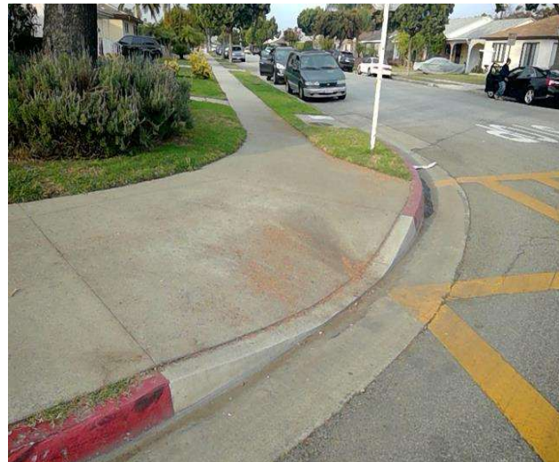
Curb Ramp : Bottom Landing Slope
