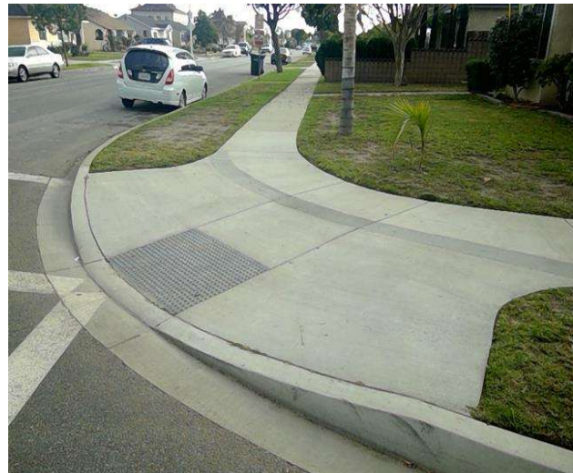
Curb Ramp : Bottom Landing Slope
