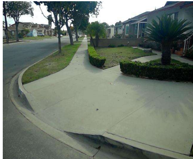
Curb Ramp : Bottom Landing Slope
