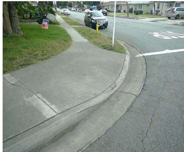
Curb Ramp : Bottom Landing Slope
