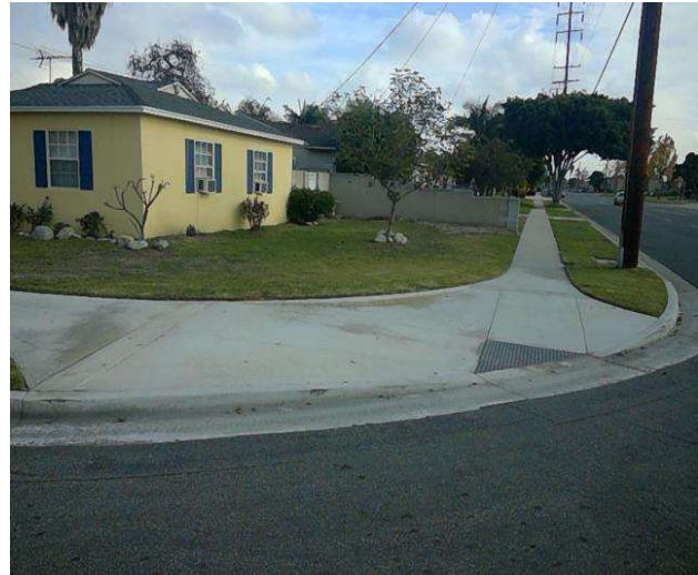
Curb Ramp , Landings and Transitions : Bottom Landing Slope
