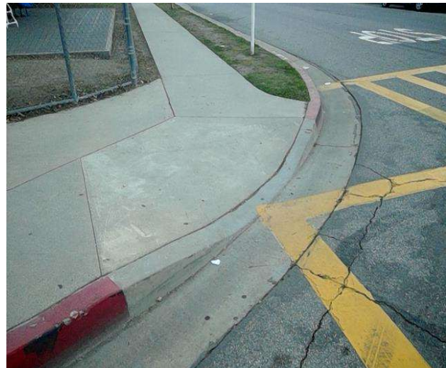
Curb Ramp : Bottom Landing Slope
