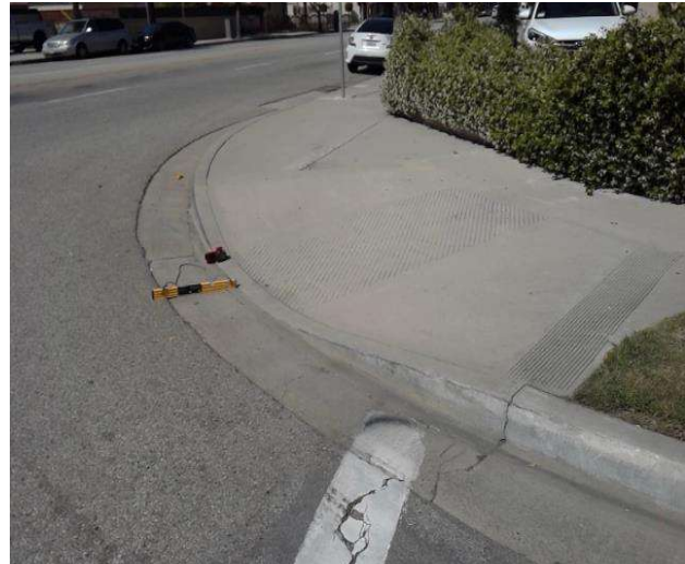
Curb Ramp : Bottom Landing Slope
