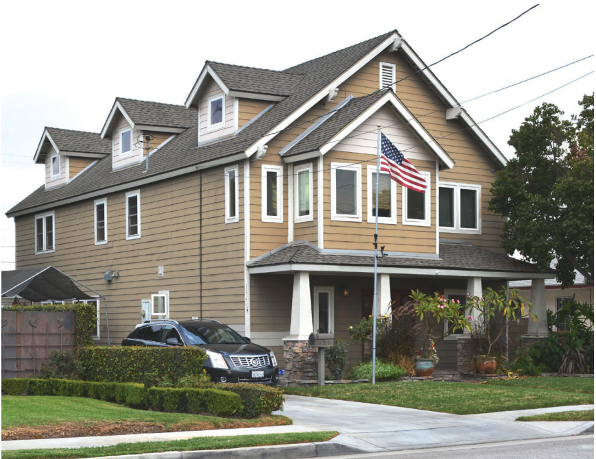
FIGURE 29: Side-facing windows at second stories should not exceed fifteen (15) percent of the aggregated side yard-facing façade area.
