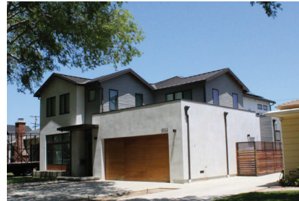
FIGURE 13: The inconsistent roof forms (flat versus gabled), materials, and styles, exhibited on this example from another Southern California city, results in a non-characteristic garage addition that diminishes the value of the existing home.
