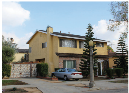
FIGURE 11: This example from another Southern California city does not utilize the same materials, ornamentation, and detailing on the side yard-facing façades.
