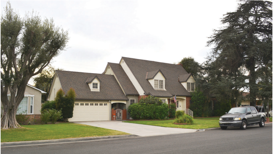
FIGURE 25: This home utilizes single-story characteristics such as incorporating dormers and encasing the first and second story under a singular roof.
