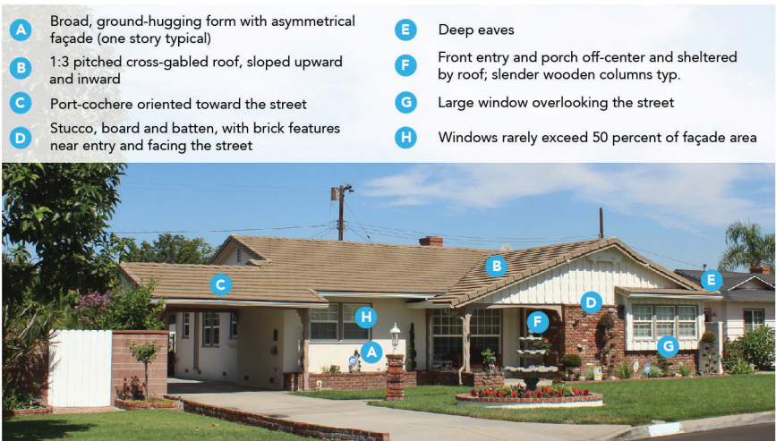
FIGURE 2: Ranch Style (Note: Porte-cocheres are subject to setback standards per Section 9312.08 of the Downey Municipal Code)
