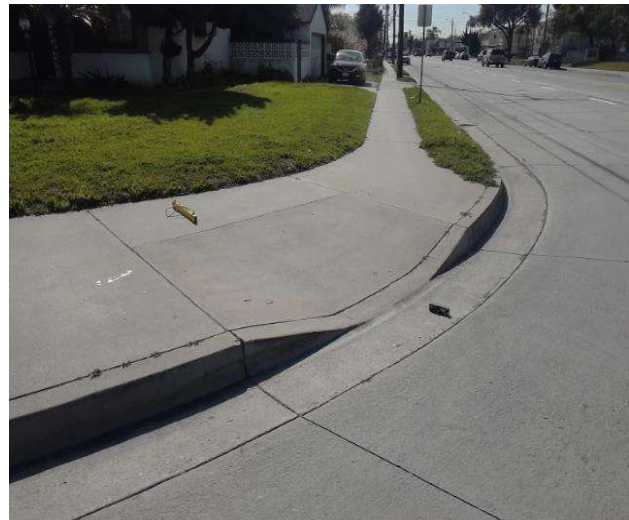
Curb Ramp : Bottom Landing Slope
