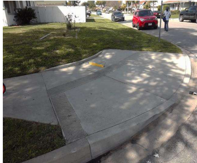
Curb Ramp : Bottom Landing Slope
