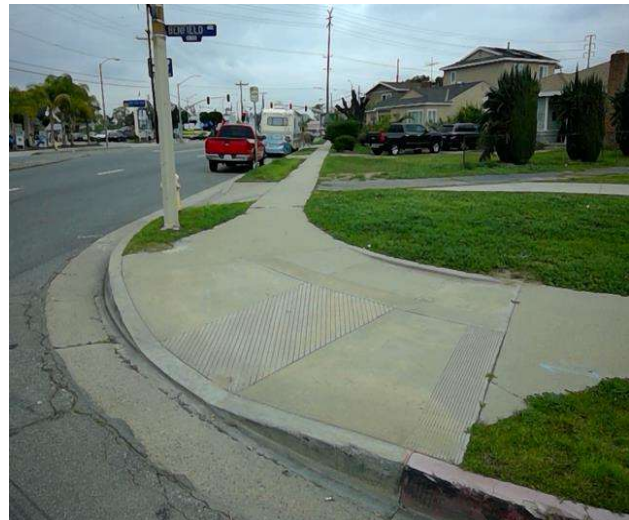
Curb Ramp : Bottom Landing Slope
