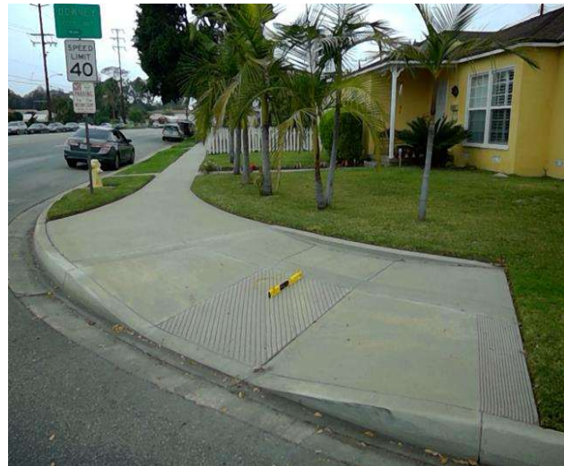
Curb Ramp : Bottom Landing Slope
