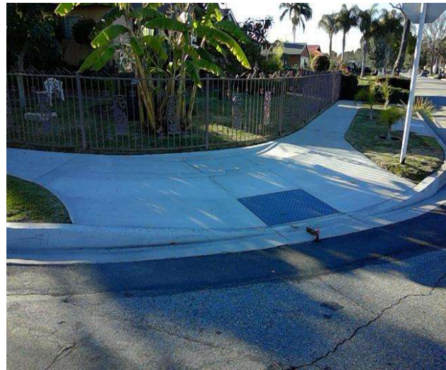
Curb Ramp : Bottom Landing Slope
