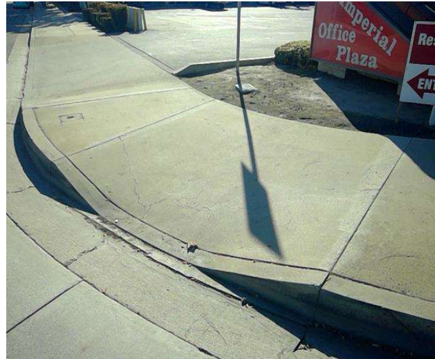
Curb Ramp : Bottom Landing Slope
