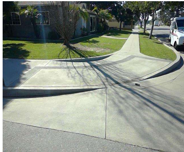
Curb Ramp : Bottom Landing Slope
