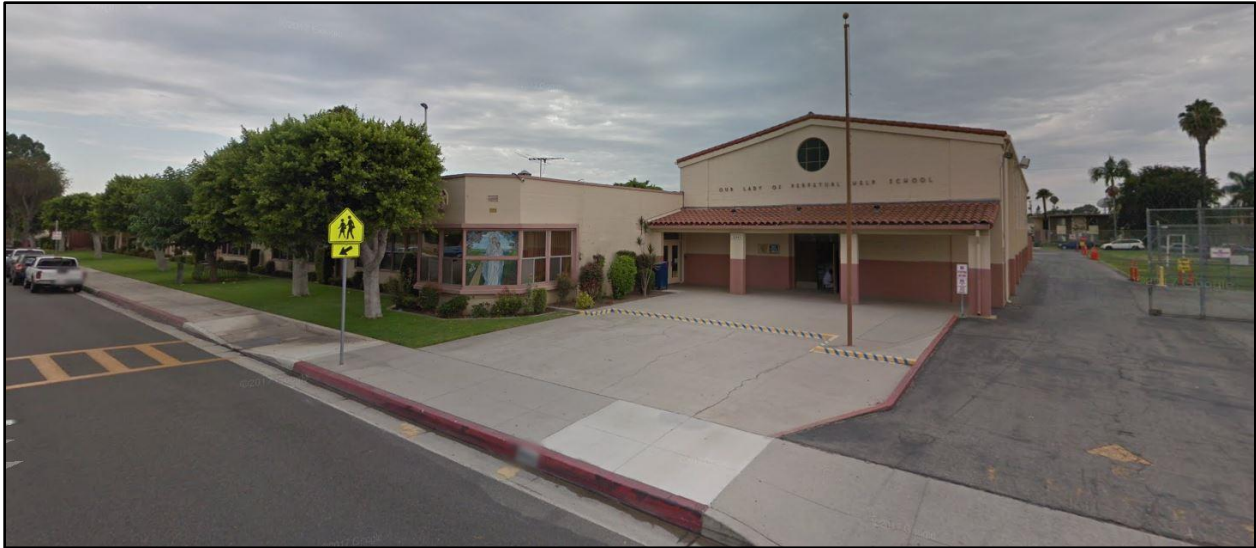
Site Photograph (from Downey Avenue)
