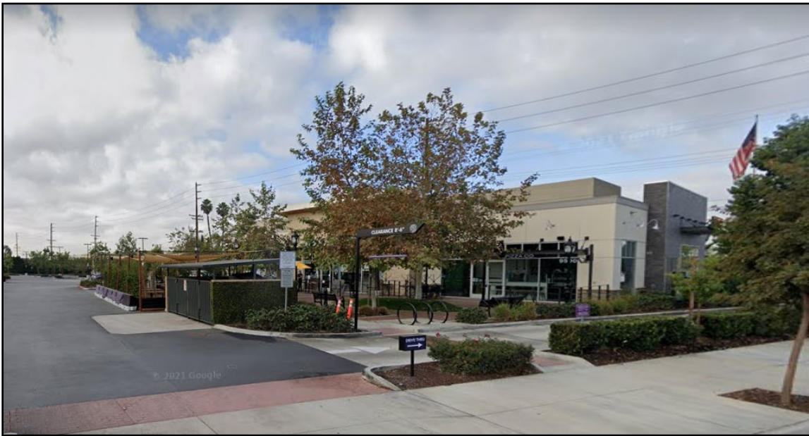
Existing North Elevation from Gallatin Rd.
