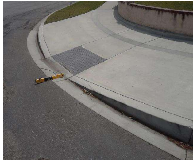
Curb Ramp : Bottom Landing Slope
