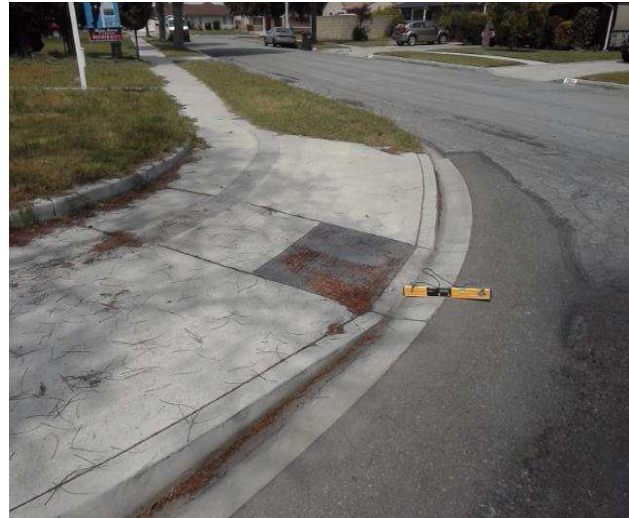
Curb Ramp : Bottom Landing Slope
