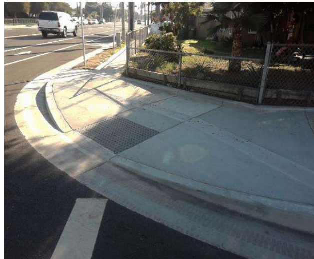
Curb Ramp : Bottom Landing Slope
