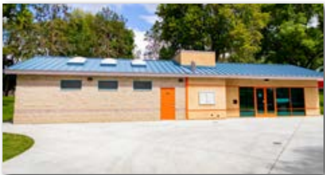
Dennis the Menace Park - New Community Building
