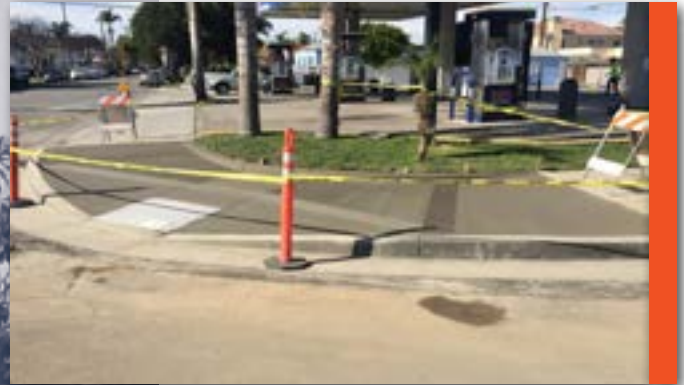
Paramount Blvd Median and Pavement Rehabilitation
