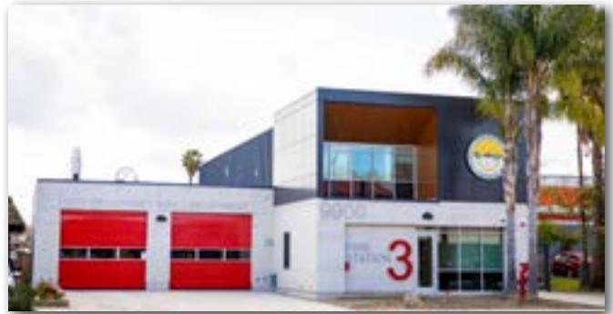
New Fire Station No. 3
