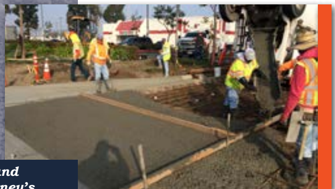
Firestone Blvd Median and Pavement Improvements
