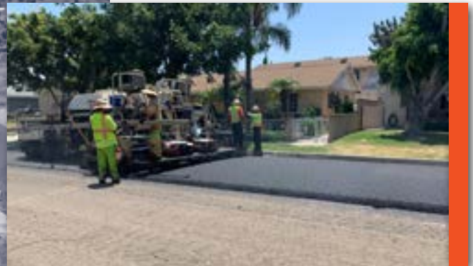
Residential Streets Pavement Rehabilitation
