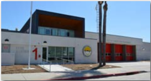
New Fire Station No. 1
