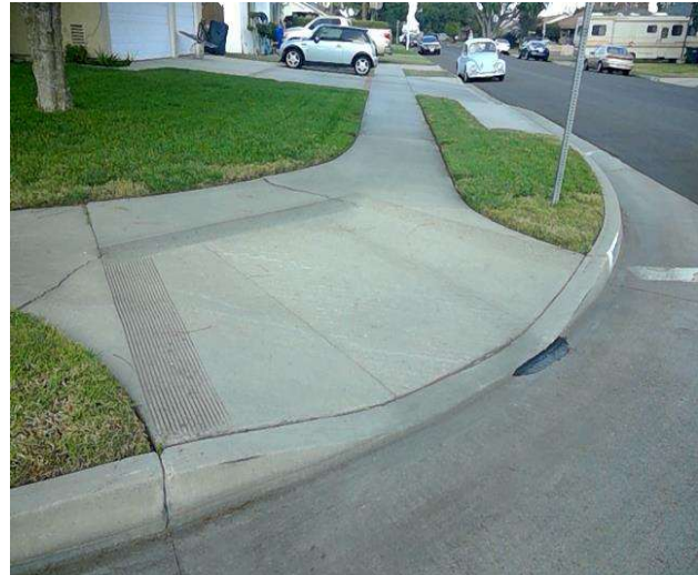
Curb Ramp , Landings and Transitions : Landing Accumulates Water - Wet Conditions
