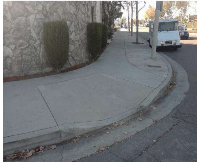
Curb Ramp : Bottom Landing Slope
