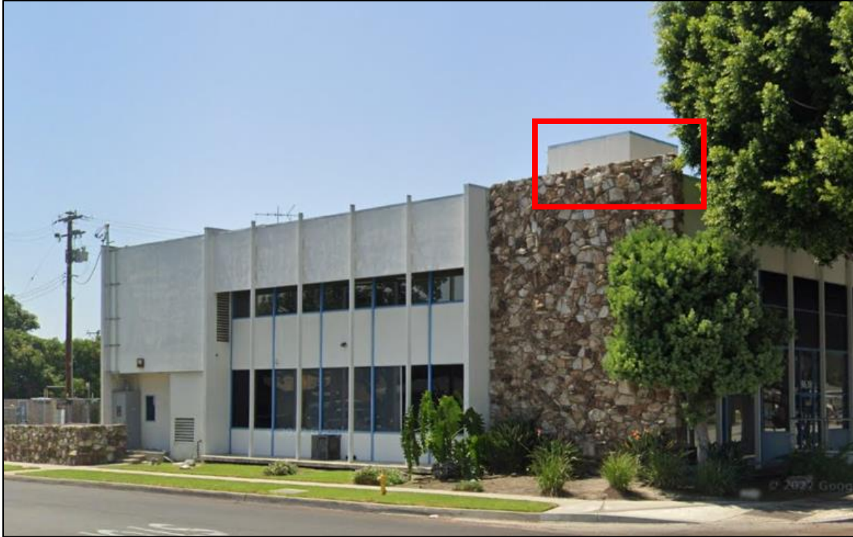
View of building
