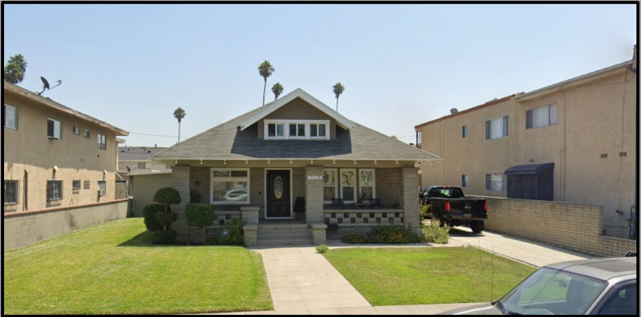
Existing Front Elevation from La Reina Avenue
