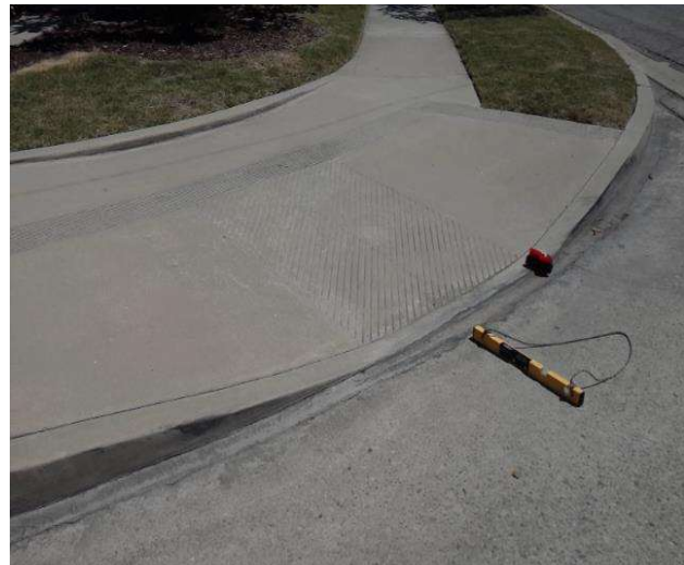
Curb Ramp : Bottom Landing Slope
