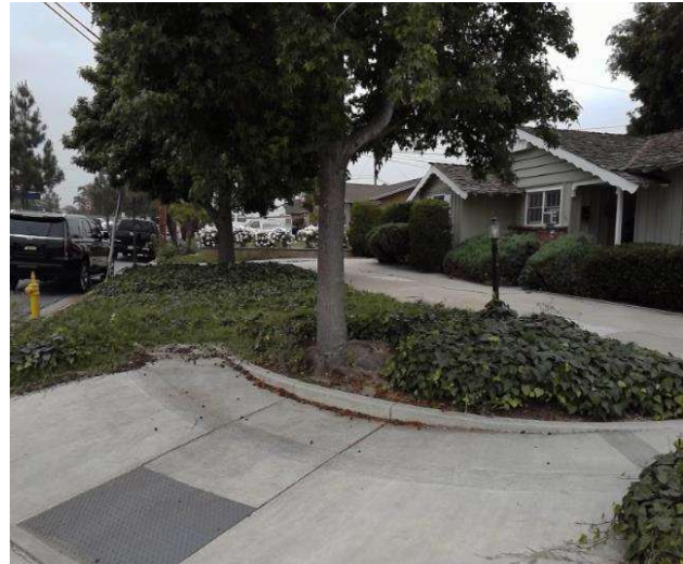
Curb Ramp , Landings and Transitions : Top Landing Right Side Clear Length - Parallel Curb Ramp
