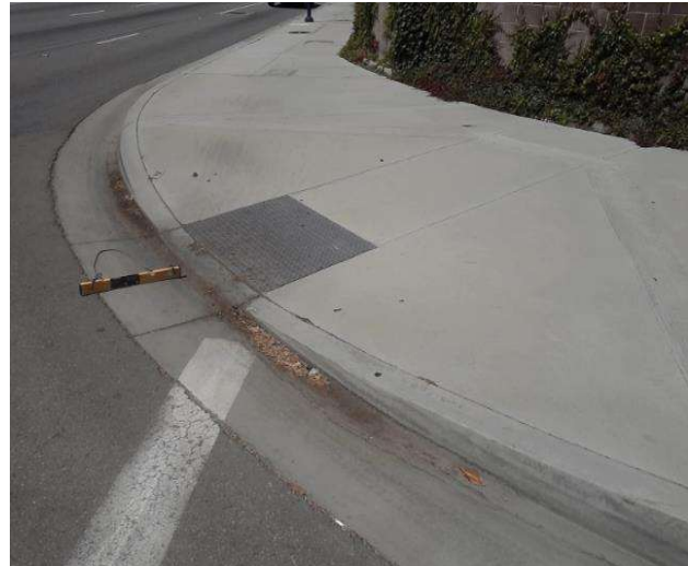
Curb Ramp : Bottom Landing Slope
