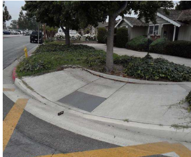
Curb Ramp : Bottom Landing Slope
