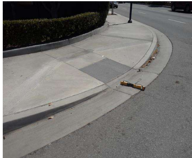
Curb Ramp : Bottom Landing Slope
