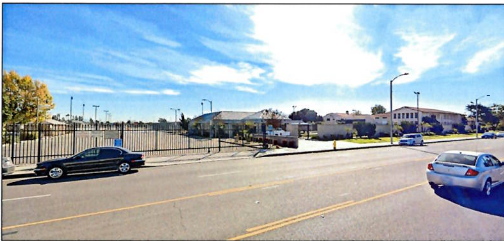
West view of subject property along Brookshire Avenue
