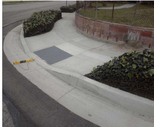
Curb Ramp : Bottom Landing Slope
