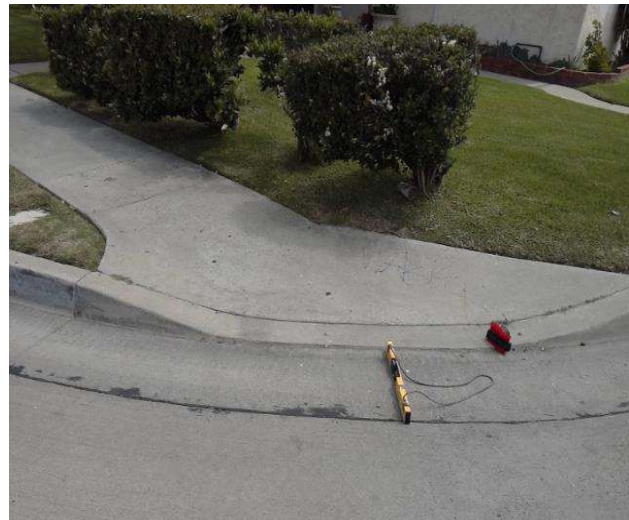
Curb Ramp : Bottom Landing Slope
