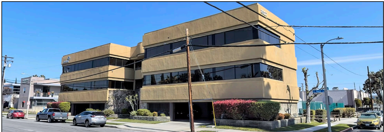
Existing Site Conditions
