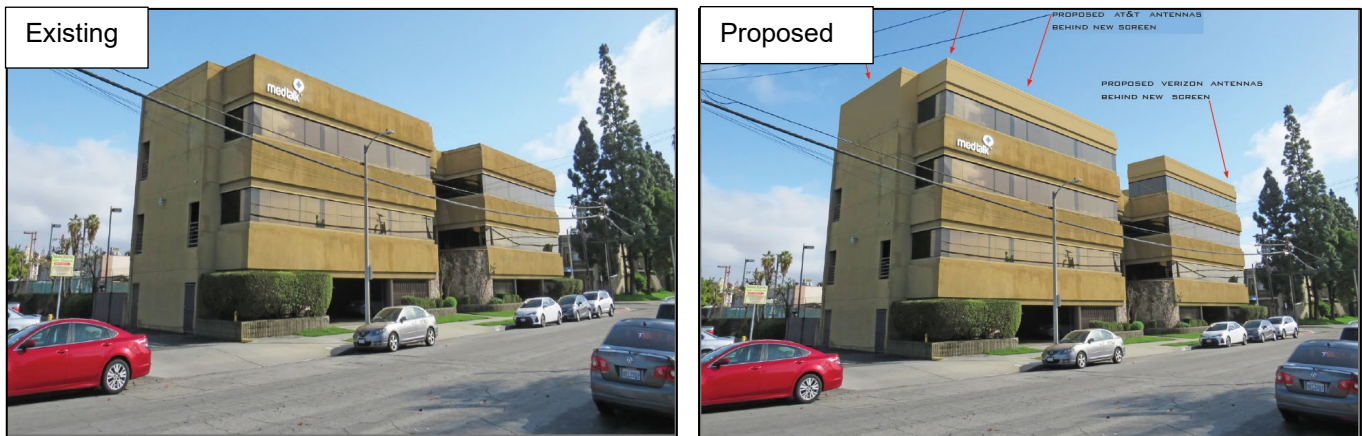
Southern section of the roof screening off Dolan Avenue
