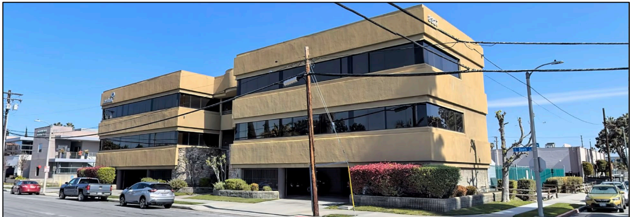
Existing Site Conditions
