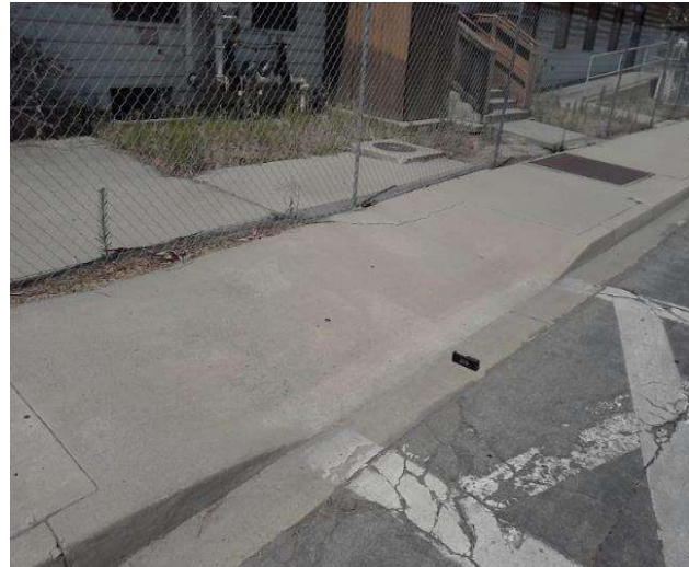
Curb Ramp : Bottom Landing Slope
