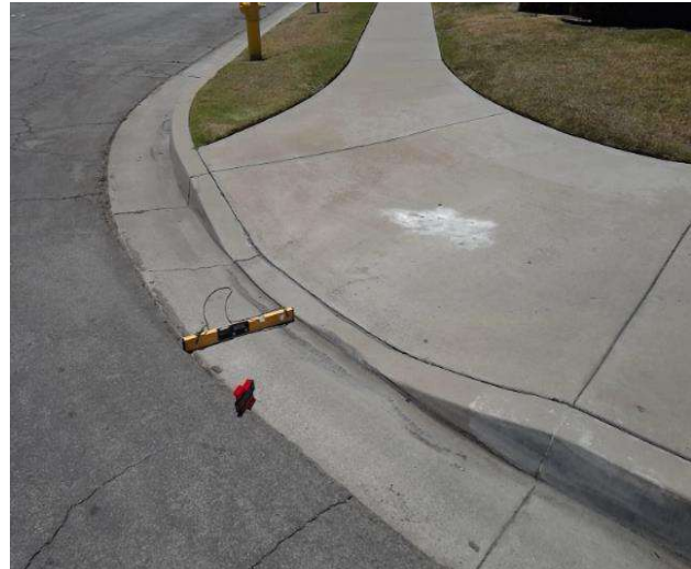
Curb Ramp : Bottom Landing Slope
