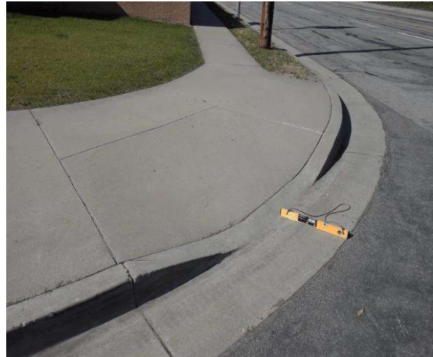
Curb Ramp : Bottom Landing Slope
