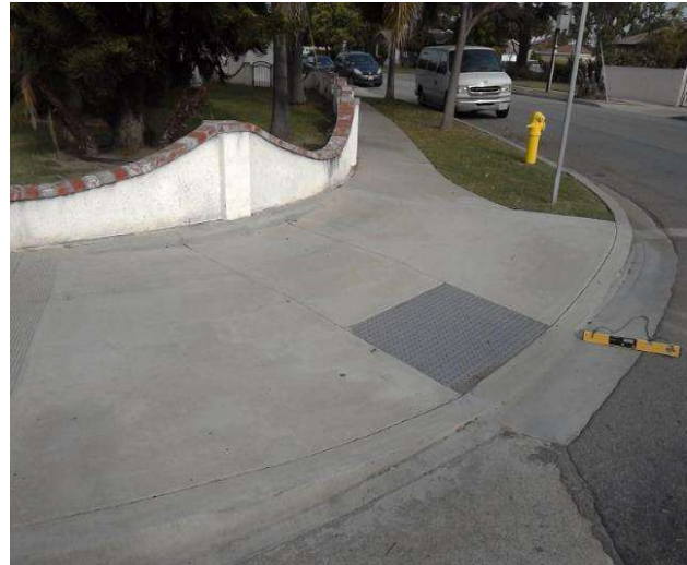
Curb Ramp : Bottom Landing Slope
