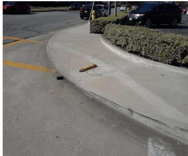
Curb Ramp : Bottom Landing Slope
