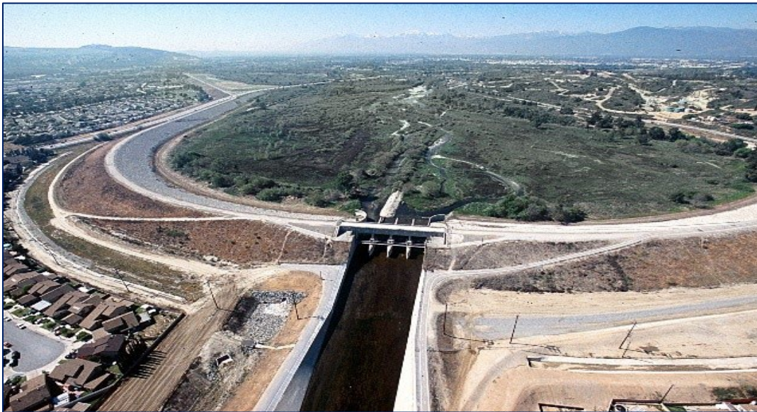
Figure 3.7: Aerial View of the Whittier Narrows Dam
