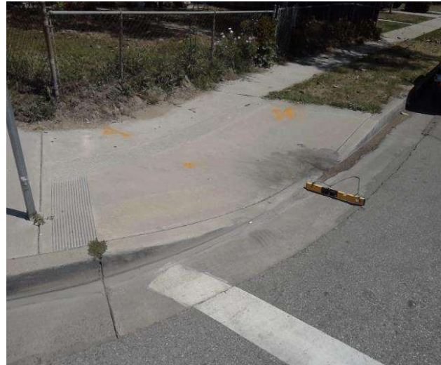
Curb Ramp : Bottom Landing Slope
