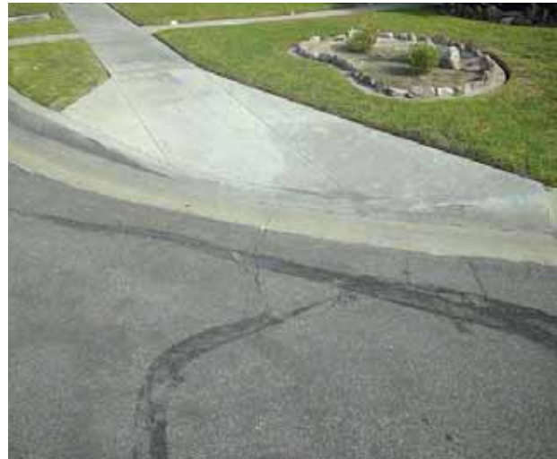
Curb Ramp : Bottom Landing Slope
