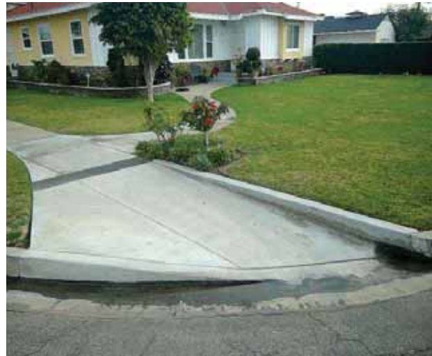
Curb Ramp : Bottom Landing Slope
