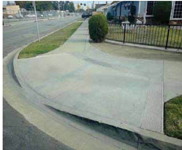
Curb Ramp : Bottom Landing Slope
