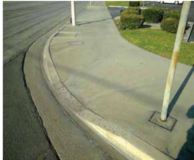
Curb Ramp : Bottom Landing Slope
