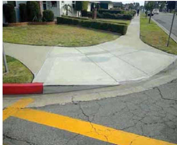
Curb Ramp : Bottom Landing Slope
