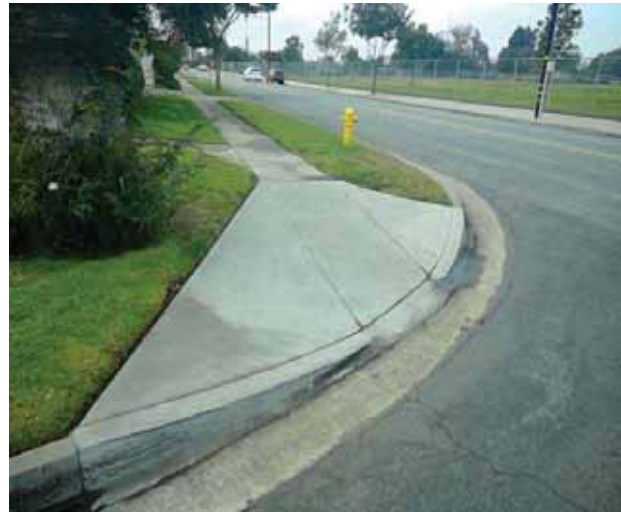
Curb Ramp : Bottom Landing Slope
